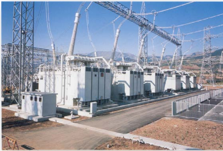
High-voltage power transformers (credit: Mitsubishi Electric)
